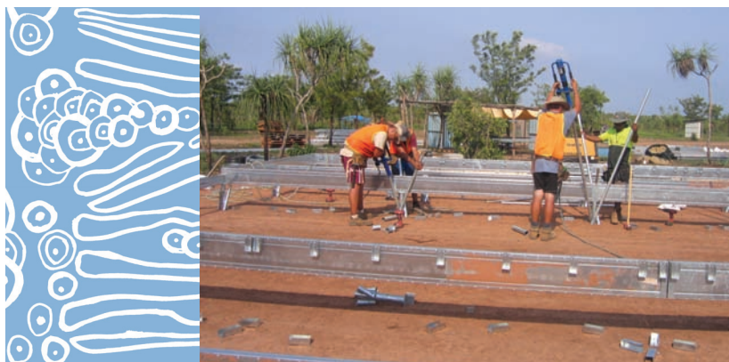
Wadeye outstation project construction site PHOTO Indigenous Business Australia
